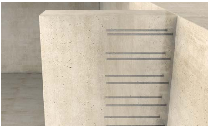
Horizontal wall connection
